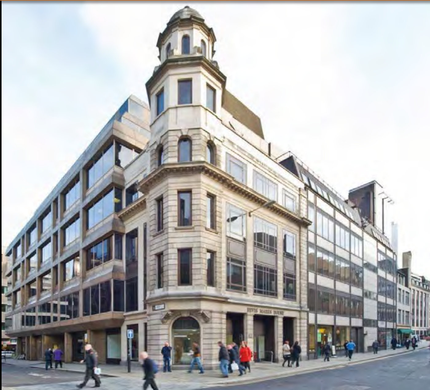
Existing corner of Goring Street and Bevis Marks
